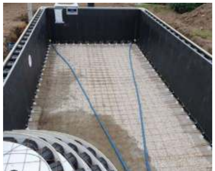
3. ASSEMBLING THE STRUCTURE AND REINFORCEMENT
